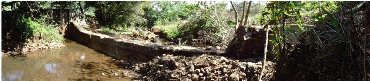
Lawai Stream Dam Diversion 812
