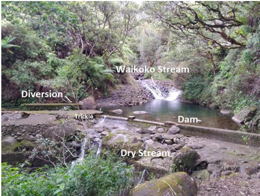
Above: Waikoko dam and diversion, Nov. 27, 2022.
