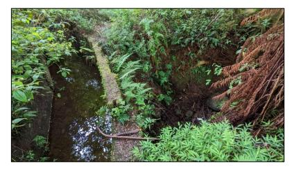
At one site along the ditch, I observed a spillway at a location where there was no natural stream channel upslope of the ditch, but there was a deep gully eroded immediately downslope of the ditch (see inset photo at left). I estimate this gully to be 10 feet deep, and it was clearly formed by water flowing through the spillway notch in the concrete ditch wall. The notch has slots for a wooden "pani board' or flashboard, but without the board in
