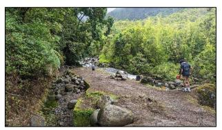
The Ili'ili'ula-North Wailua Ditch was filled in with sediment near the intake at Wai'ale'ale Stream during the site visit (see inset photo), so no measurable flow was being diverted from the stream into the ditch. The headgate in the ditch was fully boarded just down-ditch of the return flow "throw-out" which means that any water diverted from the stream into the ditch at higher flow should be blocked by the headgate and rerouted back to the stream channel through the
