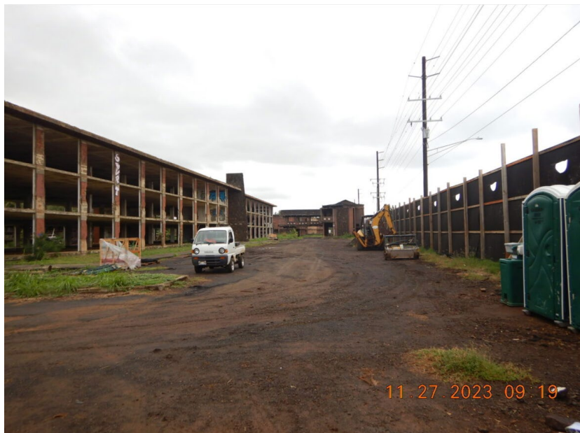
Photograph 14: View, facing north, of the road located between Building 1 and Kuhio Highway. Note the dust fence, heavy equipment, portable toilets, and handwashing station located in the enclosed area. Also, the road is covered with a layer of dirt, gravel and sand. The road is being used for vehicle and equipment to traverse the Site (see photograph 15). Photograph taken by Rande Tubal on November 27, 2023.
