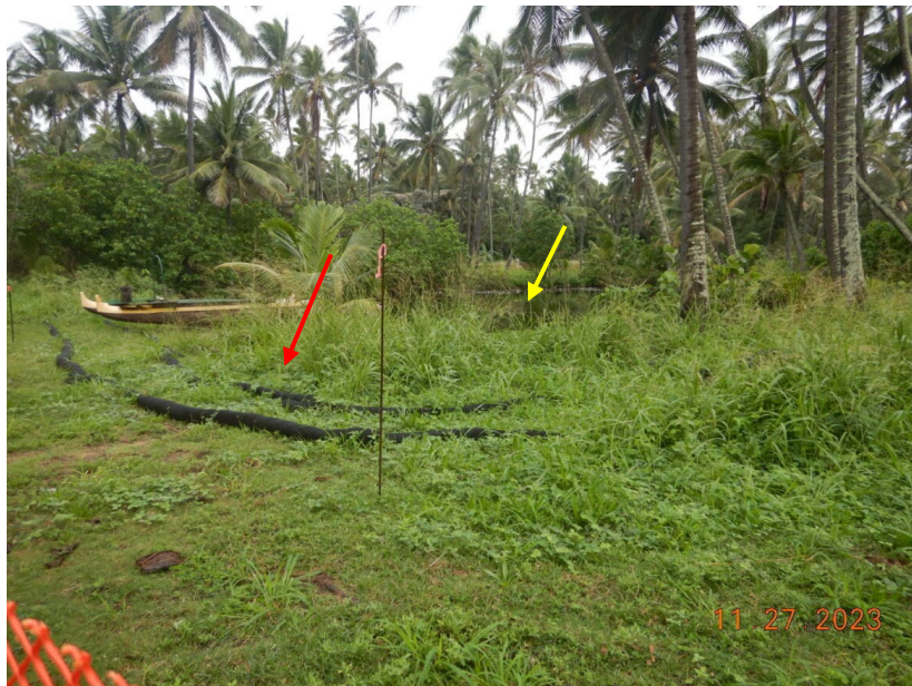
Photograph 18: View, facing northwest, of the southern end of the fishpond (yellow arrow). Note the double layer of filter socks placed around the fishpond (red arrow). Photograph taken by Bobbie Teixeira on November 27, 2023.
