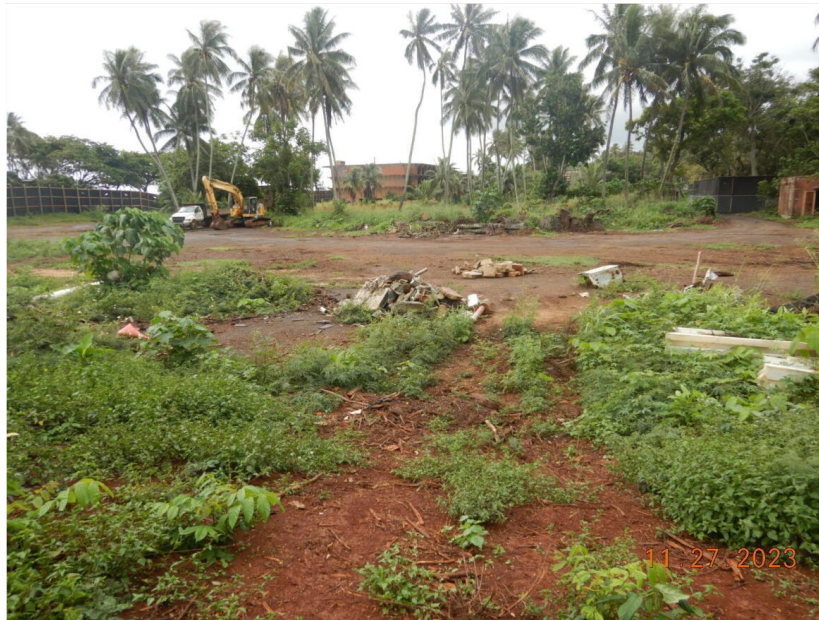
Photograph 17: Wide view, facing southwest, of northern portion of Parcel 7. Note the heavy equipment and piles of construction debris placed throughout the parcel. Also note that this portion of the parcel was cleared of numerous coconut trees (refer to Image 5, Photographs 19-20). Photograph taken by Bobbie Teixeira on November 27, 2023.
