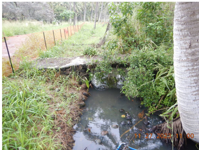
Photograph 6: View, facing north, of the State-owned Kawai iki ditch. Note the vegetation and debris present in the ditch. Photograph taken by Randee Tubal on November 27, 2023.
