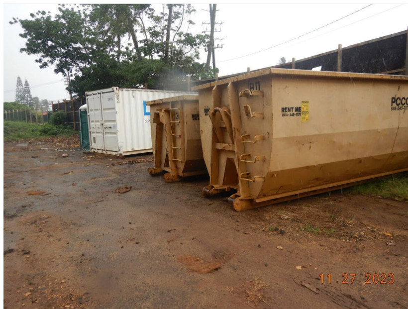
Photograph 16: View, facing northeast, of the asphalt road covered with dirt and sand, located between Building 1 and Kuhio Highway. Note, portable toilets, storage containers, and waste bins located in the enclosed area. Photograph taken by Bobbie Teixeira on November 27, 2023.
