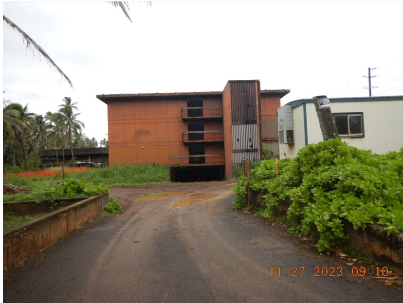
Photograph 13: Wide view, facing north, of Building 1. Note the construction trailer located to the right of the photograph. Photograph taken by Rande Tubal on November 27, 2023.
