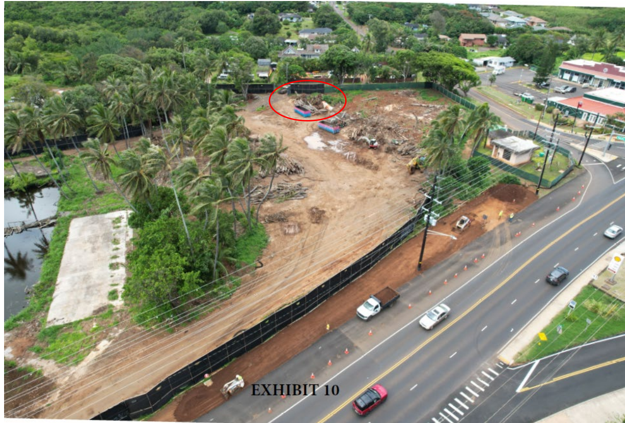
Image 5: Copy of “Exhibit 10” provided in RP21 Coco Palms’ response to the NAV-RFI. This image depicts an aerial view of the cleared area and construction debris at the Site. Note that the actual area cleared of vegetation is greater than the area depicted in the Image 4 showing the trees intended for removal. Also note the piles of root balls (red circle), stockpiles of construction debris, exposed soils, and heavy equipment present at the site.
